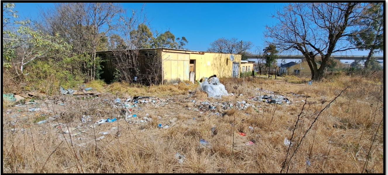
Figure 7: Abandoned building within the proposed project site.
